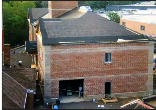
Police Station Construction
